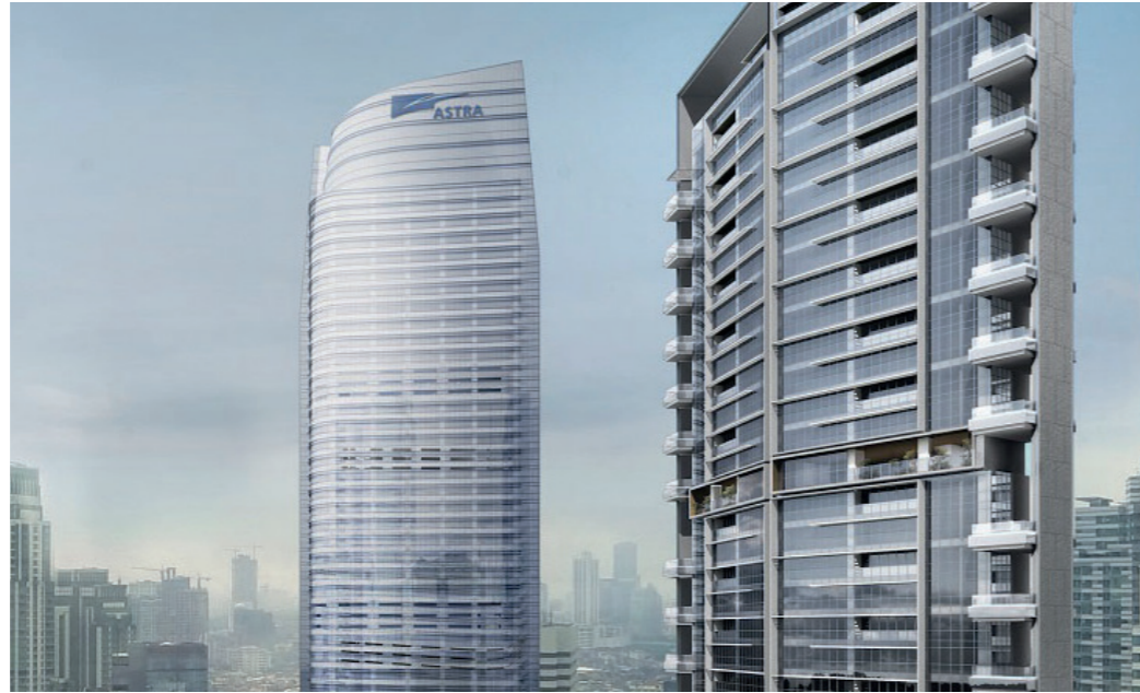
Menora Astra Tower, Jakarta, Indonesia (LEED Platinum anticipated)
